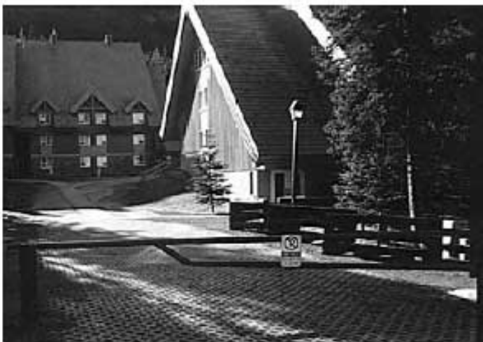
Figure 8. Emergency access lane for fire trucks
