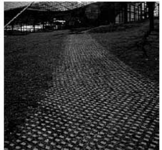
Figure 7. Service access lane
