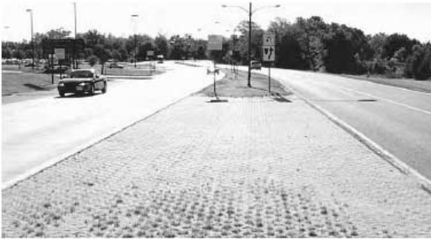
Figure 6. Roadway median crossover
