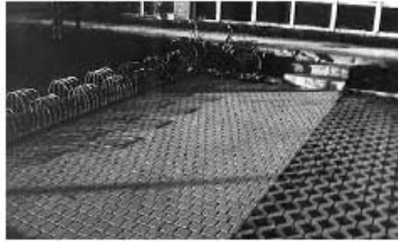
Figure 15. Solid pavers used for bicycle parking and pedestrian access.
