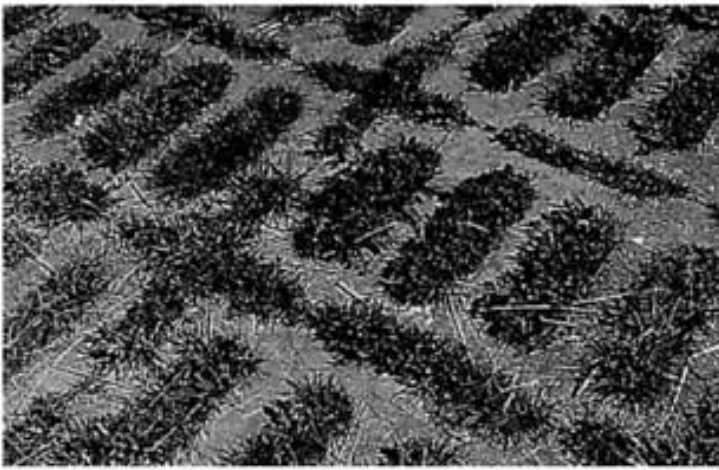
Figure 1. Grids first used in Germany in 1961 for overflow parking were building blocks placed in the ground. They emerged from the need to cool cities and decrease stormwater runoff.
