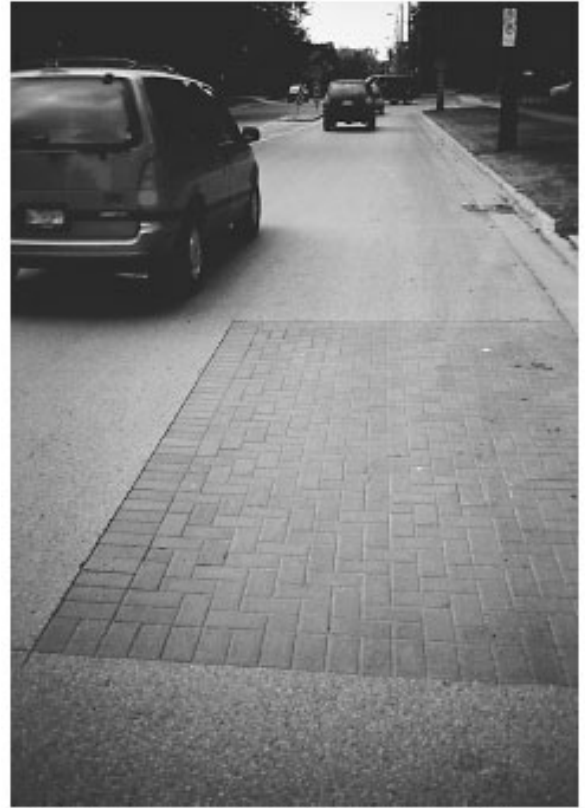
Figure 8. Utility cut repair in a residential area in London, Ontario.
