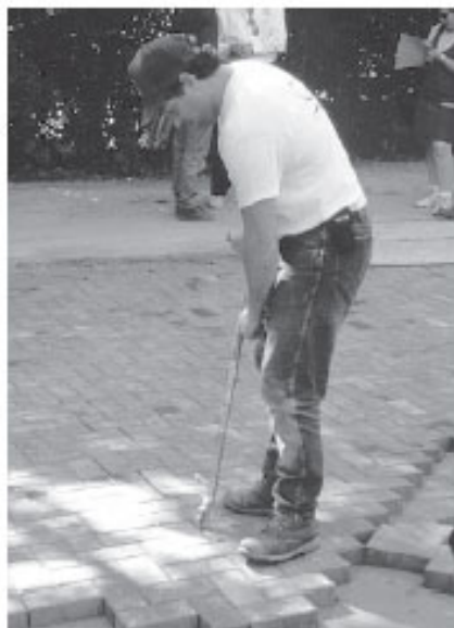
Figure 13 (Left). Adjusting joint spacing and alignment. Figure 14 (Right). Second and final compaction of the pavers. The first compaction occurs after the pavers are placed (no sand in the joints). The second compaction works the sand on pavers into the joints. This process causes the pavers to interlock.
