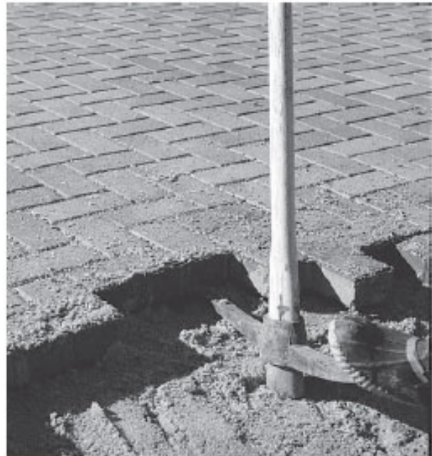
Figure 6. Prying out the remaining pavers
