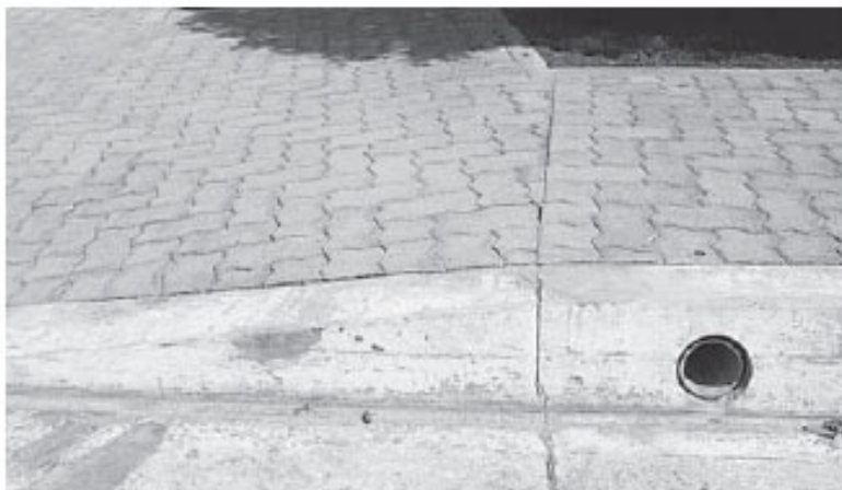
Figure 3. Ramp pavers changing angle.
