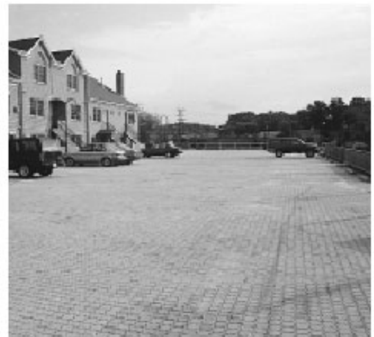
Figure 2. Concrete pavers serve vehicular traffic and parking over a concrete parking structure next to a residential development.
