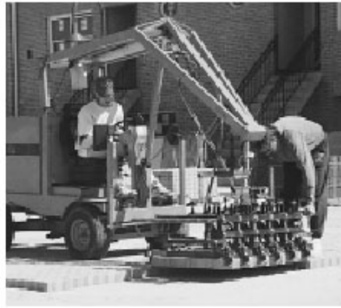
Figure 19. Mechanical equipment used to install concrete pavers on a roof deck.
