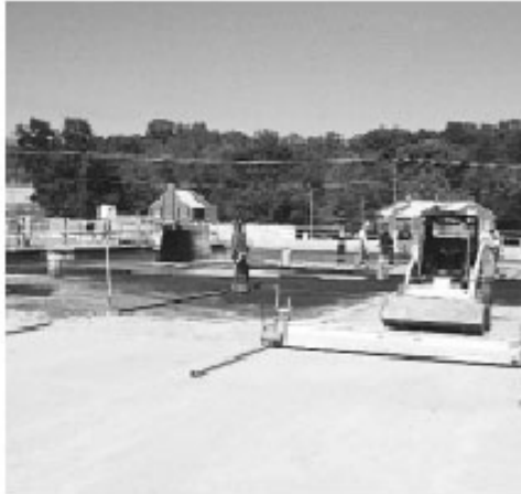
Figure 18. A mechanical screed used to level bedding sand on a roof parking deck project.
